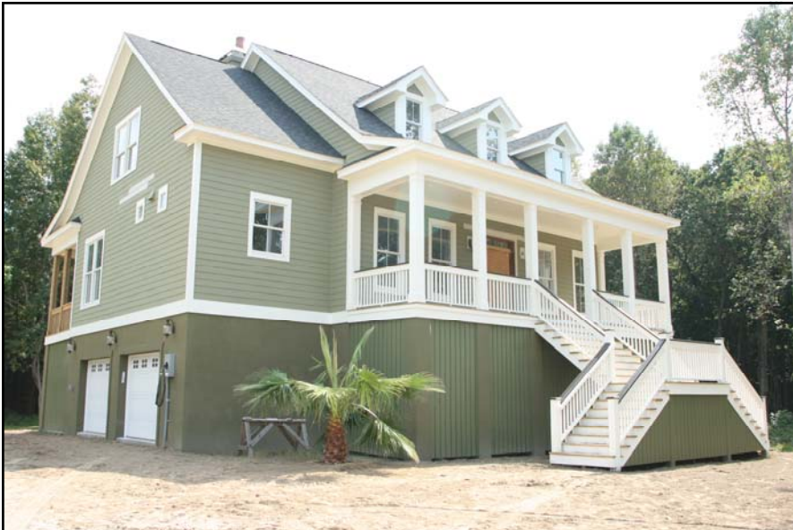
Prior to completion of landscape
